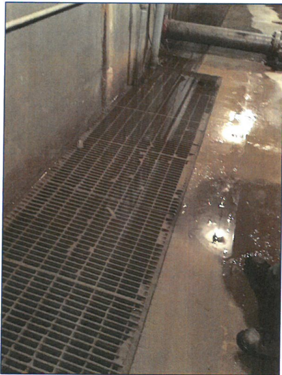
Flooded Sumps in the Basement of the Reeds Creek Pumping Building
